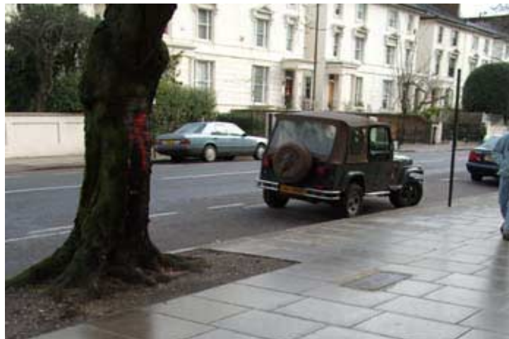
Perfectly re-laid slabs couldn't hide the evidence!
