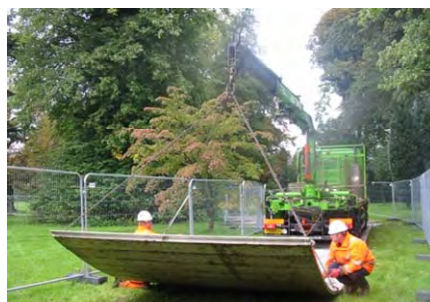
Laying temporary tracking
